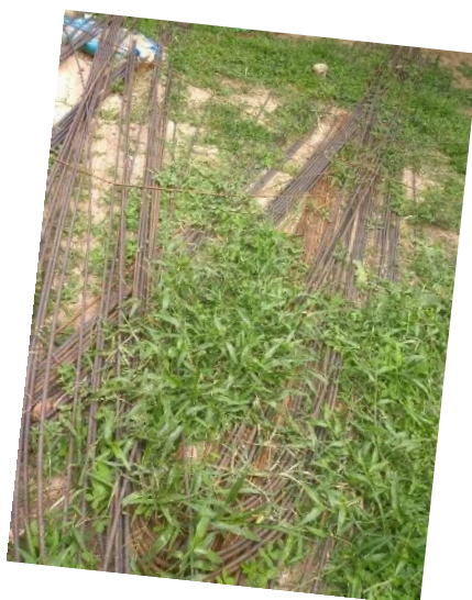
The foundation for the first part of the wall is ready
